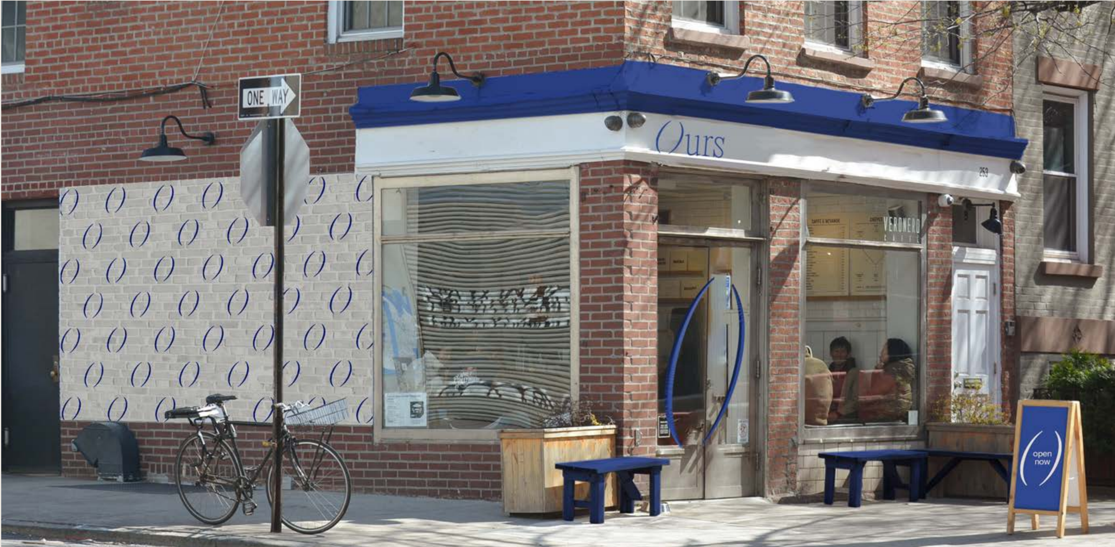
Integrate the storefront design rules to local neighborhoods. See: 253 Wythe Avenue, Williamsburg, Brooklyn
